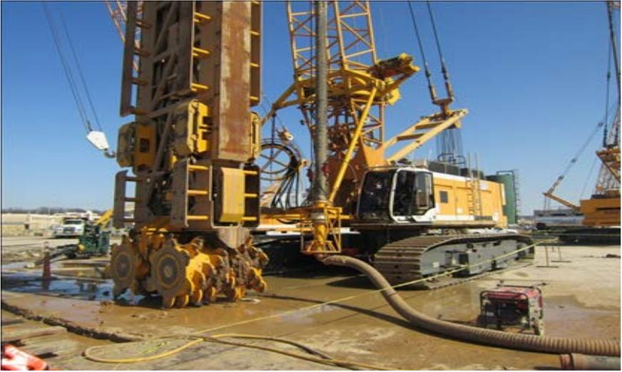
Construction of the Cutoff Wall Demonstration Section initiated in April 2017. The purpose of the demonstration section is to confirm construction methods prior to commencing production of the rest of the cutoff wall.
