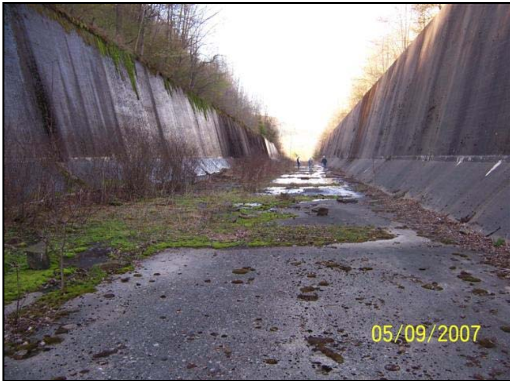
Photo 4 - A view from inside the cavernous, concrete-lined spillway looking downstream. The spillway weir would be behind and to the right of the photographer. If you look closely, three inspectors are in view which helps give perspective to the photo.
