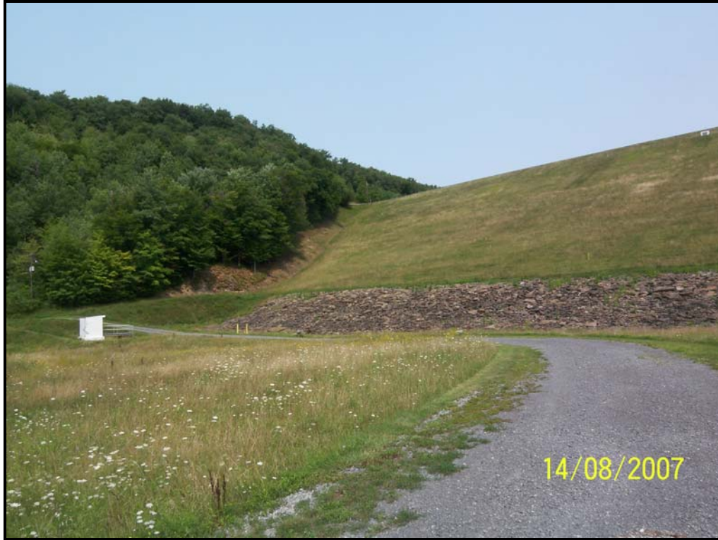
Photo 1 - A portion of the downstream face of the dam looking at the right abutment. The picture was taken from near the base of the dam. From its base to the top, the dam is 184 feet high.
