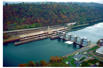
Existing Lock and Dam 4 River Mile 41.5 Originally built in 1936 Charleroi, PA
