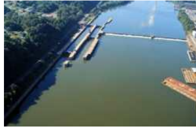
Existing Locks and Dam 3 River Mile 23.8 Originally built in 1907 Elizabeth, PA
