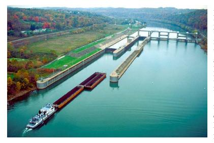
Maxwell Locks and Dam has two lock chambers, both are 720 feet by 84 feet, and a gated dam. It maintains a pool for 20.8 miles upstream to Grays Landing Lock and Dam near Grays Landing, Pennsylvania. Construction of Maxwell Locks and Dam began in 1960 and was completed in 1965. The construction of this facility resulted in the removal of old Lock and Dam 6 at Rice's Landing, Pennsylvania.
