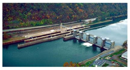
feet, the auxiliary chamber is 360 feet by 56 feet, and the dam is 535 feet in length. It maintains a pool for 19.7 miles upstream to Maxwell Lock and Dam just south of Brownsville, Pennsylvania.
