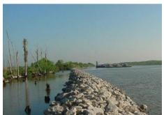
allowing for flow to flush out settled substrates and cleaning the backwaters to preserve the desired gravel substrates. This cycling of material should serve to replicate a natural river habitat more closely than the current channel conditions. This measure is primarily aimed at meeting planning objective 1. See Engineering Appendix (Appendix A), for an example of the Parallel Dike Measure.
