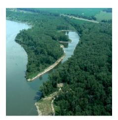
Figure 8: Exposed Parallel Dike
