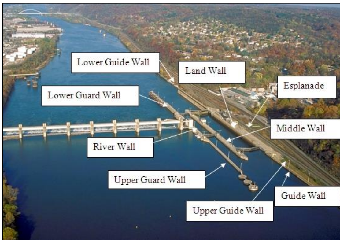
Photo 4-1: Lock Wall Component Nomenclature
