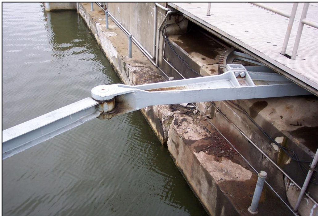
Photo 4-5: Miter Lock Gate Machinery (Arm)
